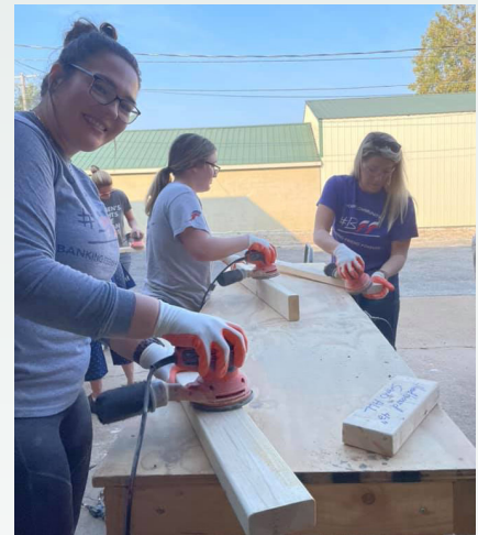
First Federal Savings Bank, Evansville
